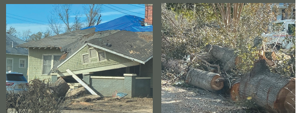
Tornado Damage in the Southeast Region After the January Tornado above
