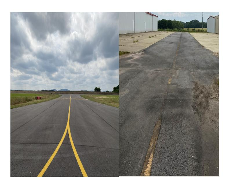
Taxiway markings are generally in <u>GOOD</u> condition. However, Taxiway markings located next to the hangars are in <u>POOR</u> condition.
